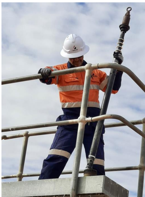
Photo 2: Bass operator retrieving a jet pump from a Worrior well
